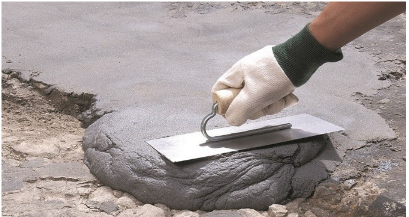
Resin based Repairs of Concrete
